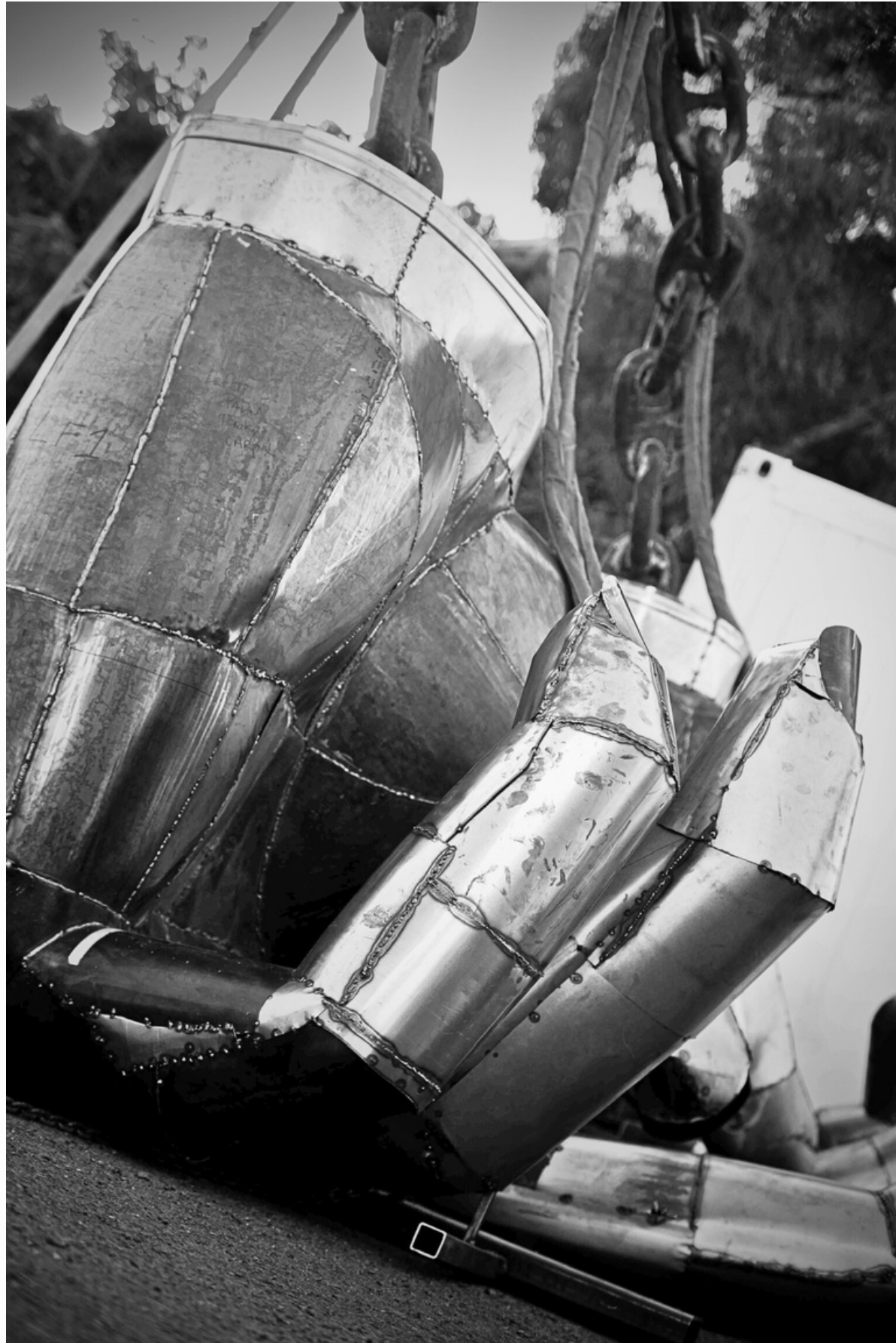
Work in progress: Build location - Petaluma, CA
